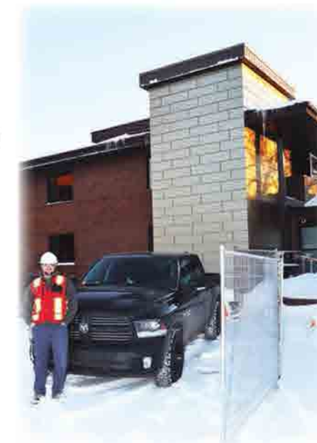
New elevator exterior entrance
